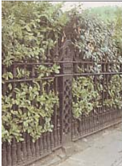
Railings, York Gate, NW1.
