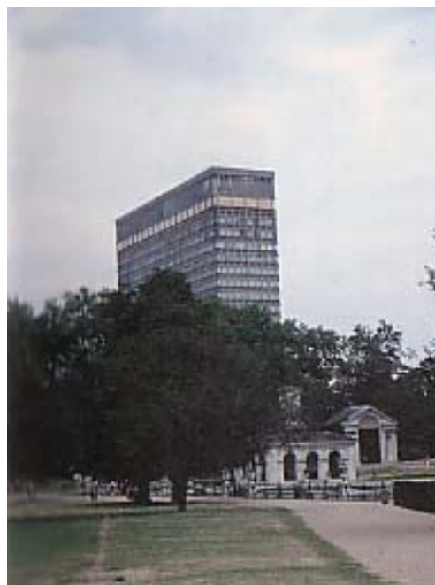
Various examples of the impact of high buildings outside Royal Parks on the landscapes and views within them.
